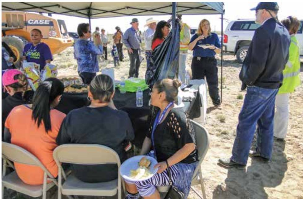
Project Engineer Charles Fiedler, with Gordon Environmental, watches as more than 40 residents and elected officials attend the groundbreaking of the Chaparral Collection and Recycling Center.
