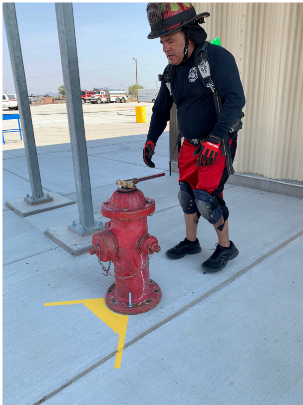
Hydrant Opening, Painted triangle- No stepping in this area
